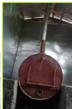
Installed heater ready for testing. Top ceiling to be covered.
