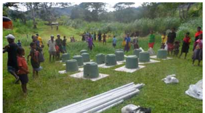
Delivery of toilet seats and bases plus fittings at Efogi village
